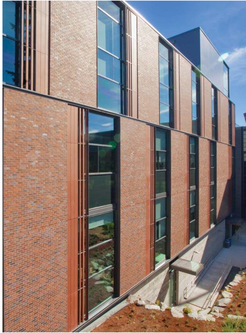
Thermafiber® RainBarrier® 45 continuous insulation (ci) was installed on the University of Washington Bothell, Discovery Hall in Bothell, WA.
