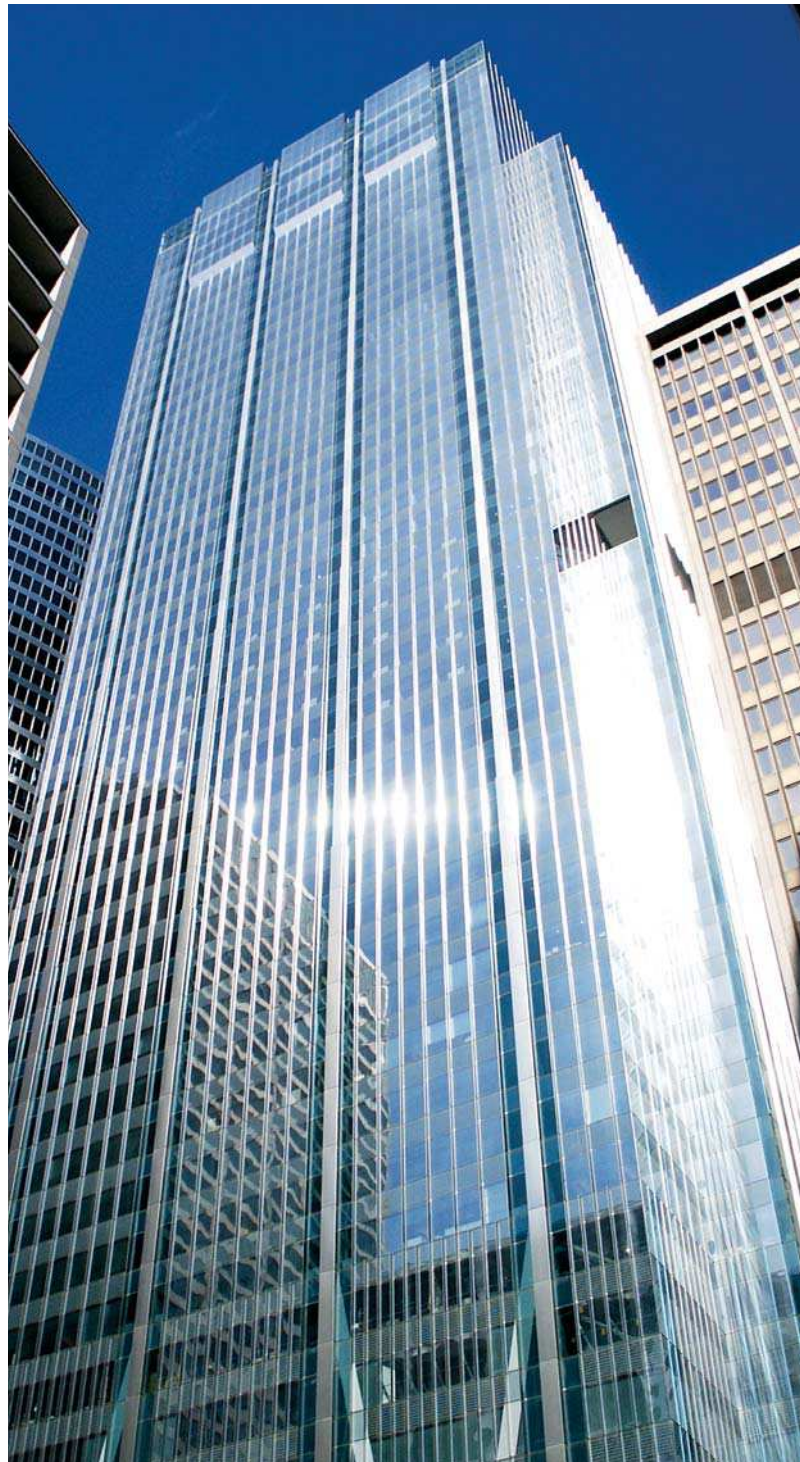
Thermafiber® Safing and FireSpan® insulations provide the critical components of the perimeter fire containment system in the 111 South Wacker Building in Chicago, IL. Thermafiber® mineral wool insulation also contributed to the building's LEED® Gold Rating.
